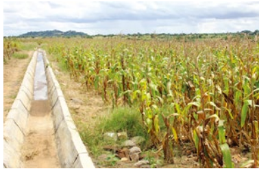
Irrigation Scheme: Zimbabwe
