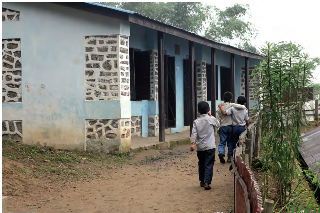
A retrofitted school building in Ilam, rebuilt after the 18 September 2011 Earthquake.
