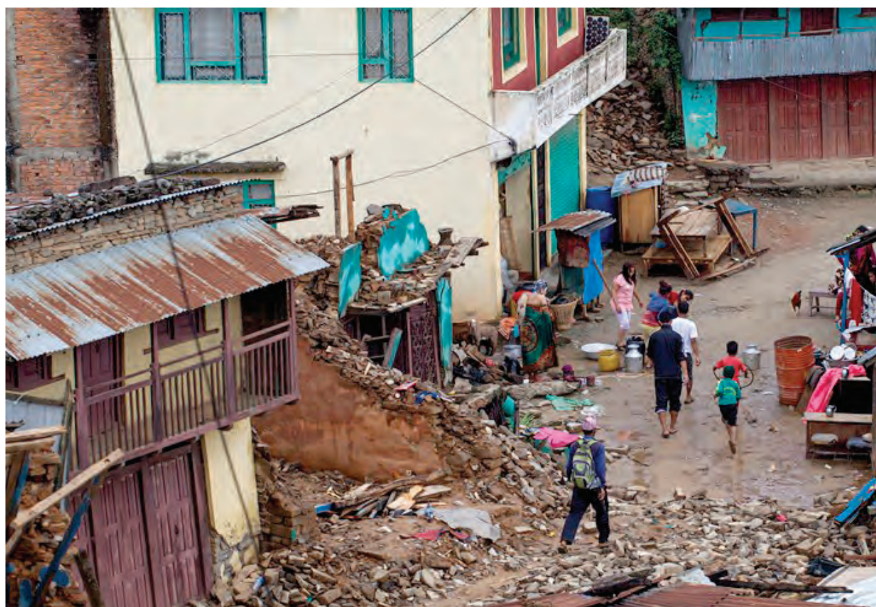
Houses destroyed during the April 25 earthquake at Rupinala village, Masel VDC in Gorkha
