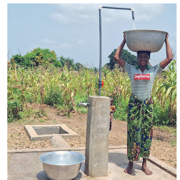
This water point in Yeldidong, Ghana, has an elevated tap to help ease the physical strain for those who carry containers on their heads.
