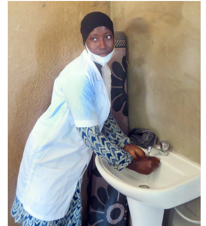
Nurse Roukaya washes her hands at a new sink in the Boulounguey Health Center. The small, community-built center has three rooms and serves 9,200 people from five villages in Niger’s Dosso region. The facility has a new water system for drinking, handwashing, and cleaning needs, as well as sanitary toilets.
