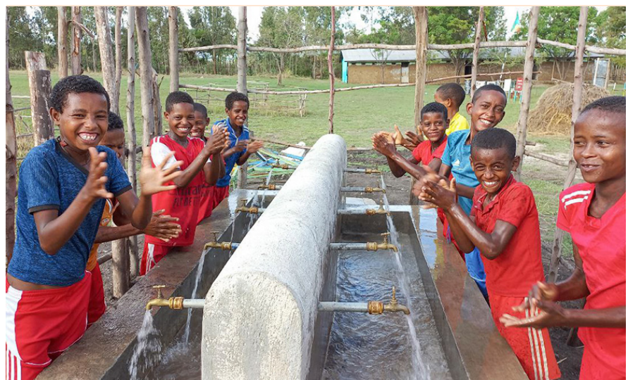
These Ethiopian schoolboys can wash their hands and drink clean water at the new taps installed at their school.
