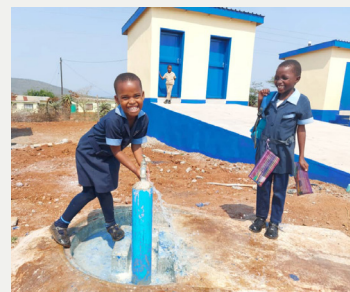
Ramps at taps and latrines provide easier access for students in Eswatini who use wheelchairs or walkers.
