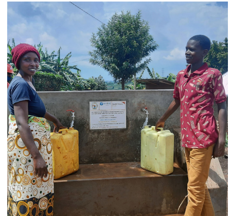
Residents of Rutare enjoy getting water from new community taps recently constructed through the support provided by donors like you.
