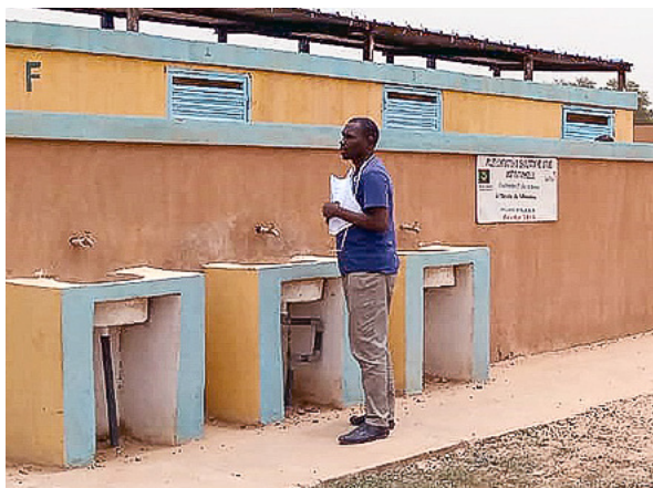
New latrine blocks at a school in Dar el Barka AP in Mauritania are sex-segregated and have handwashing stations for students.
