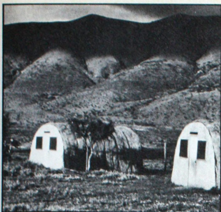
(above) Shaped like the Masai's traditional huts, these more healthful and durable homes have ferro-concrete frames and a layer of polyurethane under their grass-thatch roofs. (right) Uona is able to irrigate his garden because of the earth-filled dam built by Denny and his village team.
