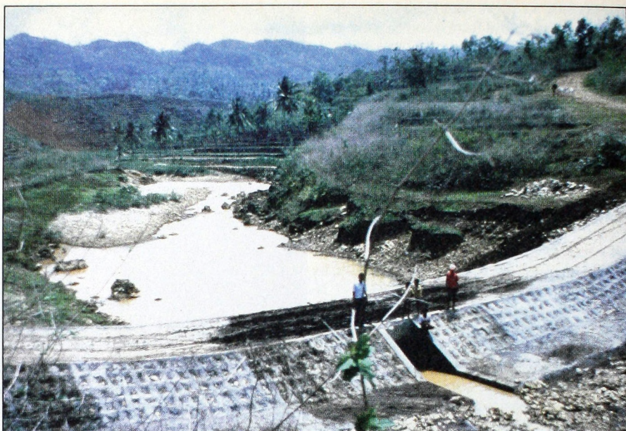
Using available building materials, Rus helps a community in the dry area of Central Java build a dam to conserve the little rainwater they get during the wet season.
