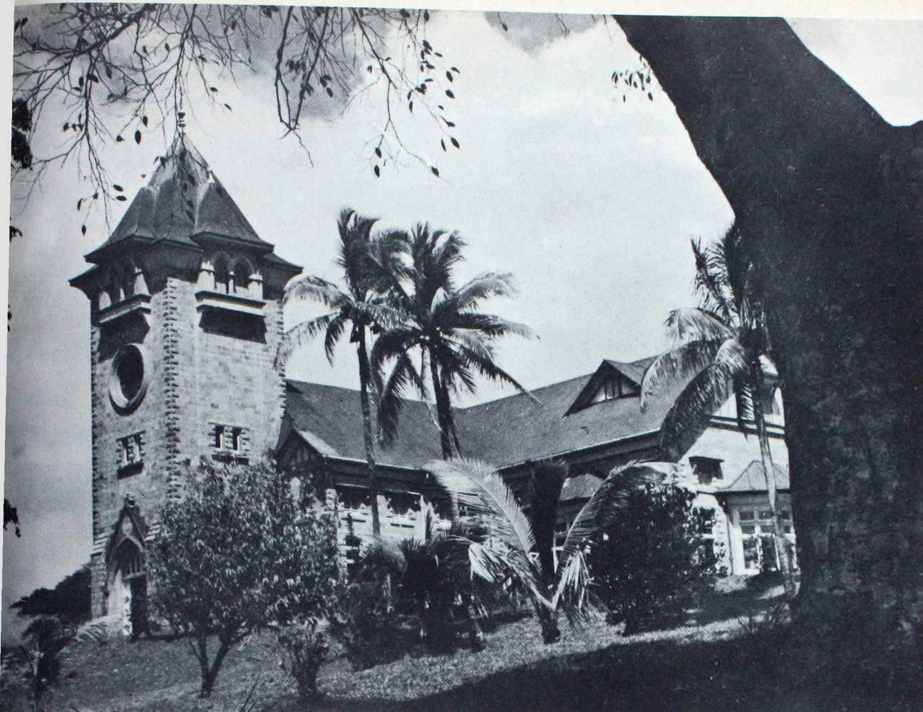
Baker Memorial Hall built by Fiji Christians at Davuilevu.
