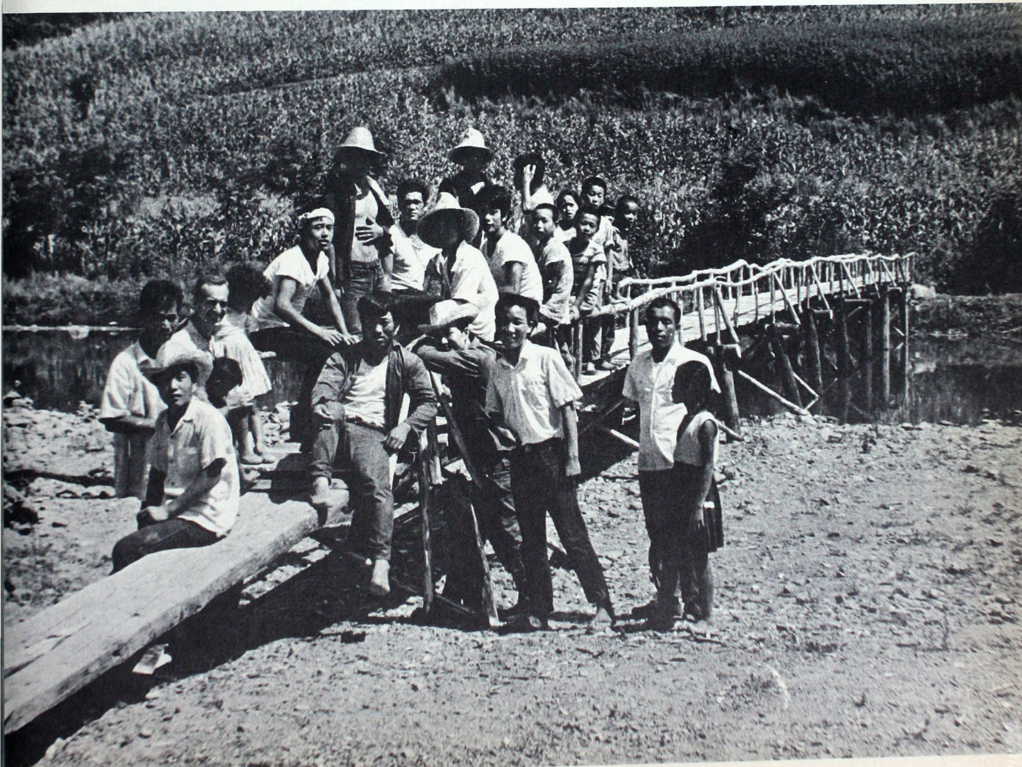
Before the rainy season, campers at Jesus Abbey and local villagers build a bridge.
