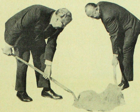
Dr. Richard C. Halverson, Acting President, and Claude Edwards, member of the Board of Directors, turn the first shovels full of earth for the construction of World Vision's International Center in Monrovia, California.
