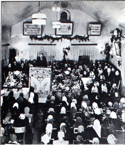
This humble sanctuary in Minsk, Russia, was confiscated by the Soviets without compensation. The hated church was banished to city's outskirts where, at great expense, an old building was remodeled. Churches are padlocked, believers imprisoned and tortured, their homes bulldozed. But fearless witnesses throughout Russia openly proclaim gospel. Many conversions, mainly youth.
